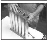
4. Insert vane and rail assembly into the ductwork and secure using standard self-drilling screws. Secure rail to ductwork per SMACNA standards.
