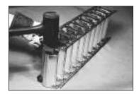
Assembly is ready to be inserted into the duct. Fasten to duct wall per the SMACNA recommendations.
