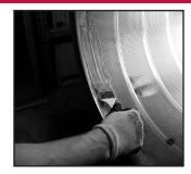
6. Seal the joint internally with PROseal® duct sealant. Brush the sealer into the joint achieving a 100% seal.
