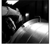
5. Continue in one direction attaching the flange to the duct 1" from the face of the flange, 10" on center around the circumference of the duct. Optional stitch welding around ECONO*flange* Double Wall to duct 10" on center. Assure stitch welds cover 50% onto duct and 50% onto flange for strong weld.
