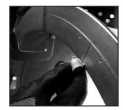
7. The break in the flange will allow a portion of the leading edge of the duct to be visible. For a better seal on medium to high pressure jobs (4" and higher) it is preferred that a short piece of Ductmate 440 gasket be applied to the face of the flange to cover the leading edge on both mating flanges. (On low pressure jobs the 440, applied to the split, can be replaced by Ductmate Neoprene gasket.)
