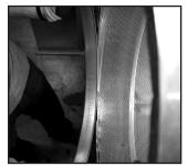
2. Start the ring by inserting the 13/4" leg inside the duct.
