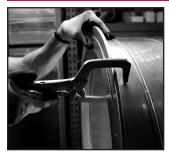
3. Seat the ring flush with the end of the duct and clamp the ring into position.
