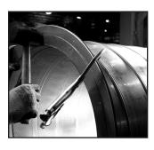
4. Begin securing the leg of the ring to the duct section at the split. Hold the flange in position by placing vise grips a few inches from the break. Begin placing a self drilling screw, spot weld, or line rivet ½" from the break.
