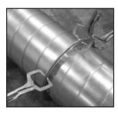
10. Clamp the mating ECONO*flange* Double Wall rings compressing the gasket until the mating rings touch.
