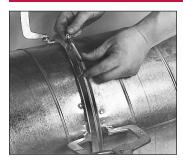
Slide closure ring over mating flanges and insert bolt.
