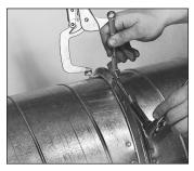
10. Tighten the bolt on the closure ring until it makes even contact around the circumference of the duct sections. Tap around joint with hammer if necessary to seat flange while tightening.
