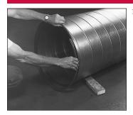
Start duct flange by inserting duct end into flange pocket at the break in the ring.
