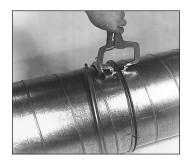
Slip outer closure ring over end of duct. Align flanges using Spiralmate alignment grips.
