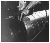
8" - 18" duct - 8" on center 20" - 28" duct - 12" on center 30" and larger duct - 18" on center d. Continue in the same direction around the duct at evenly spaced intervals, as noted below left. Place the last fastener within 1/2" of the end of the duct flange.
