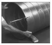
Seat flange permanently by pressing it so the leading edge of the duct is seated in the pocket of the flange and penetrates the sealant.
