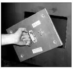
4. Insert the door into the opening at an angle and then center the door.
