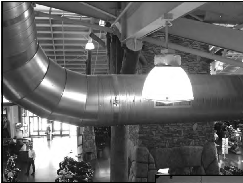
Installation of CL23-WC6 Cable Locks and WC6-CL23 wire rope.
