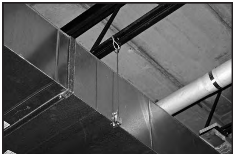
An installed Dyna-Tite KV Bracket and Duro Loop Cable
