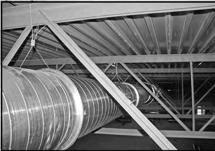
Installed CL23-WC6 Cable Locks
