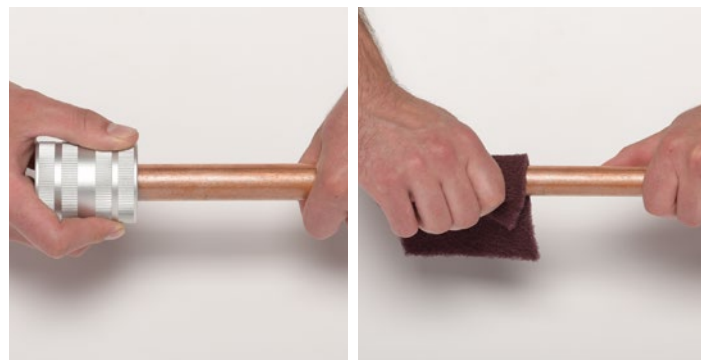
Following tube preparation steps 4 to 8 in the RLS installation instructions is important for preventing leaks.
