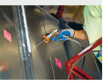
Contractors appreciate the substantial time and labor savings achieved when utilizing Carlisle HVAC's sprayable products to seal their ductwork. Carlisle HVAC offers customized Mobile Sealant Delivery Systems that have been designed to maximize production and minimize maintenance. The Carlisle HVAC Mobile Sealant Delivery Systems are designed with a customized cart to secure the pail of sealant, larger pumps to extend the life of the pump and a wide range of pressure settings and tip sizes.
