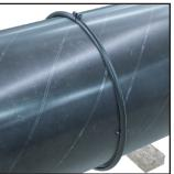
10. Tighten the bolt on the closure ring until it makes even contact around the circumference of the duct sections. Tap around joint with hammer if necessary to seat flange while tightening.
