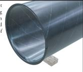
3. Begin securing the leg of the flange to the duct section by placing a pop rivet, screw, or spot weld within 1/2" of the end of the flange break. The fastener should be placed no closer than 3/4" or further than 1" from the face of the flange.
