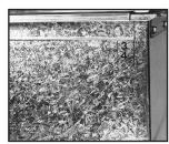
It is essential that the frame angle is fastened to the duct within ¾" of the end of the angle at each corner.
